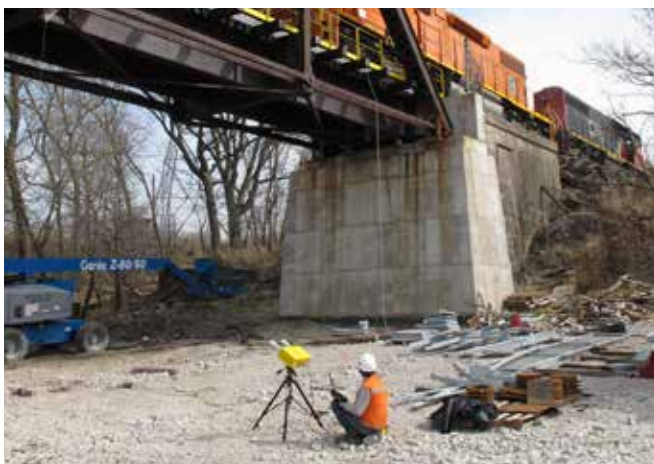
IBIS-FS monitoring an iron bridge
